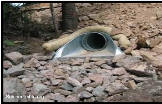
Drainage Outlet Protection
